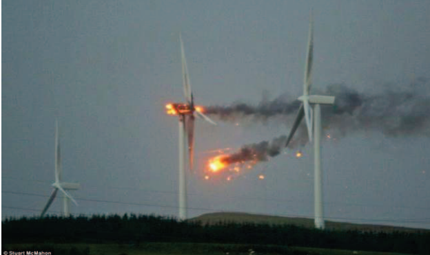
Wind Turbine Fire in Ayrshire Scotland
